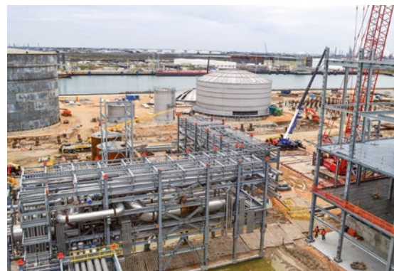
The Corpus Christi, Texas, polyethylene terephthalate plant, seen here in 2016, still isn't completed.
